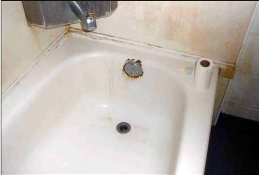
Figure 3 Intake Bathroom Detail: Bathtub
