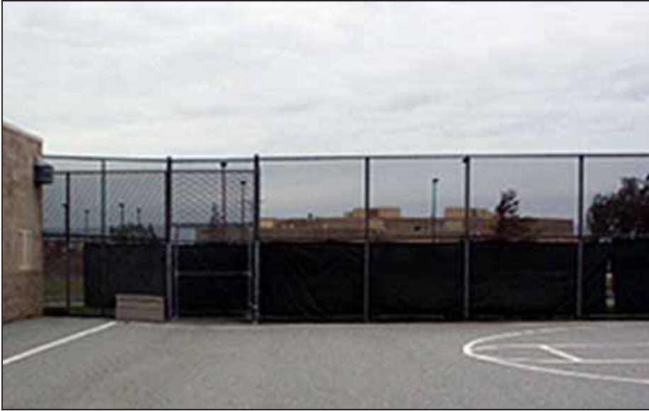
Figure 18 Back Security Fence (North side facing the County Jail)
