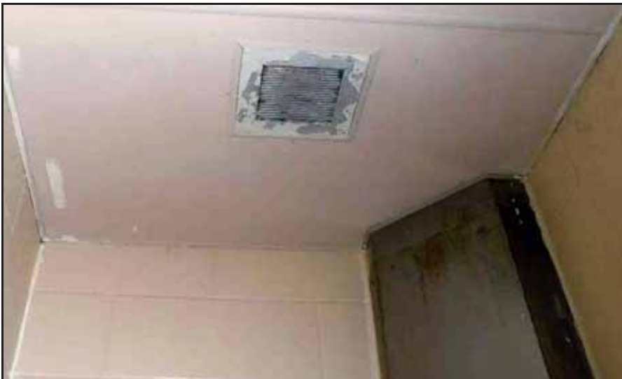
Figure 4 Intake Bathroom Detail: Shower Stall Ceiling
