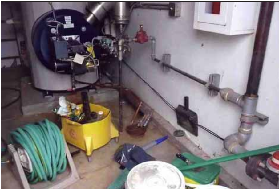
Figure 17 Storage in Boiler Room
