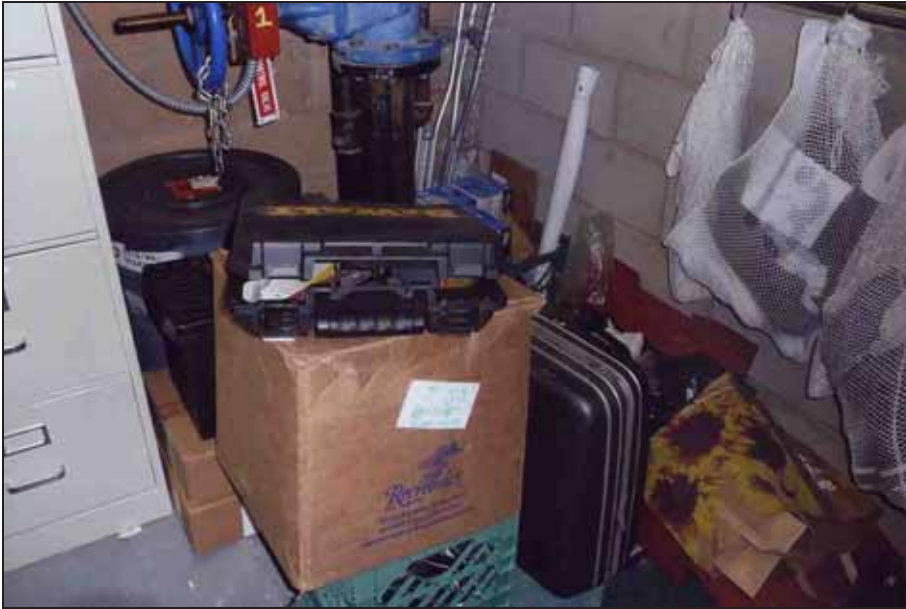
Figure 16 Storage Closet next to the Multi-Purpose Room
