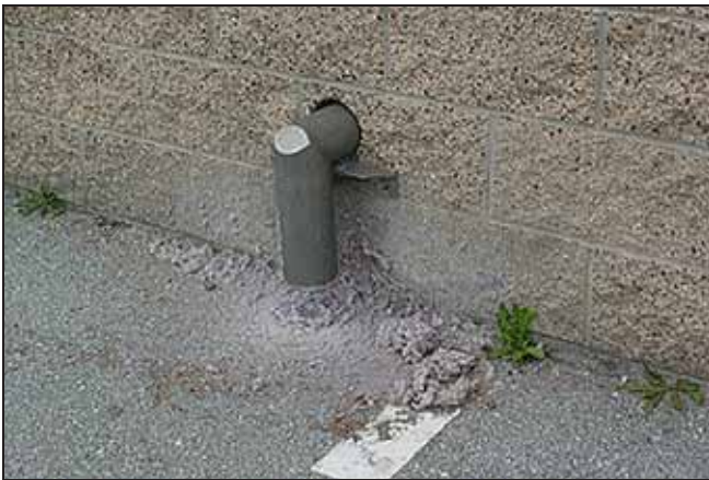
Figure 12 Laundry Room Vent Area
